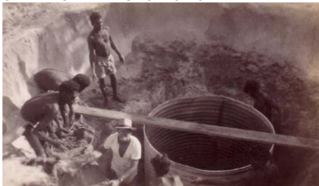
PIC043/0874: Digging the well
