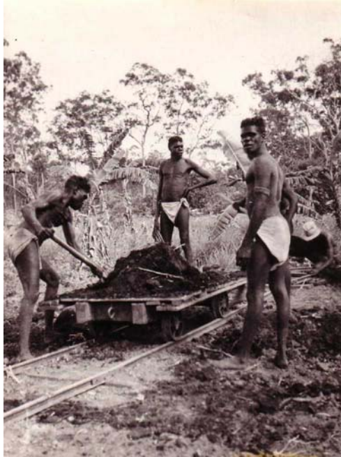
PIC043/0880: Shifting soil on tracks NANGURRMA WURRWILLIA TOPPING UP DAM BEFORE CYCLONE CAME
